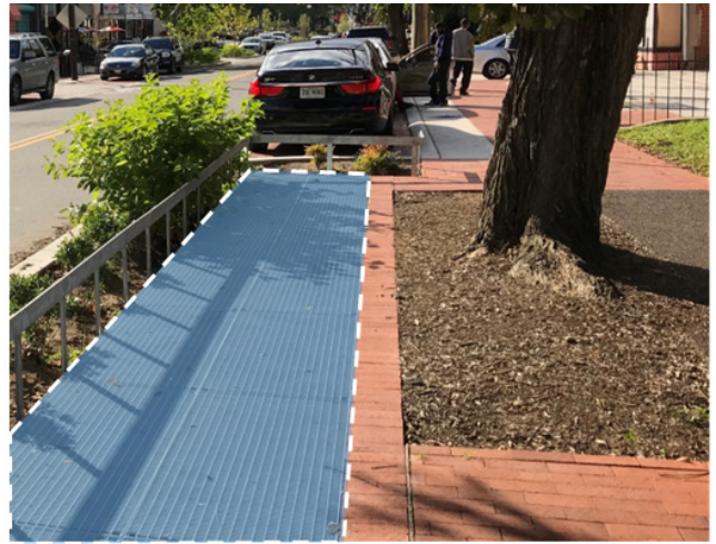
After: Elevated catwalks preserve trees and create accessible pathways
