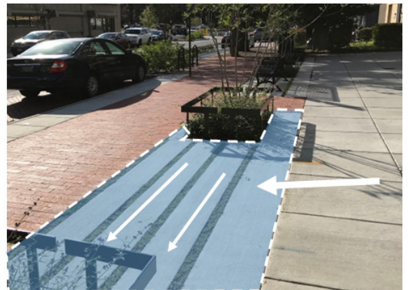
After: Landscape Infiltration Gaps (LIGs) capture stormwater to Subsurface system
