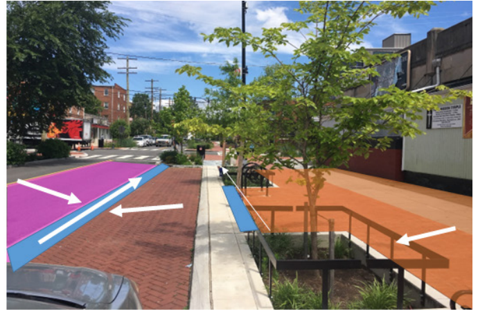
After: Crown Street Profile collects stormwater in different channels to slow and distribute flow
