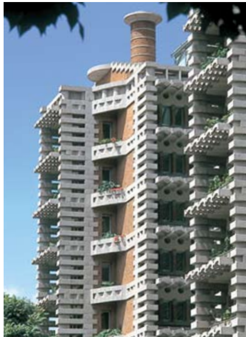
THE VENTILATION SYSTEM FOR THE EASTGATE CENTRE IN HARARE, ZIMBABWE, WAS INSPIRED BY THE VENTILATION OF TERMITE MOUNDS. THE BUILDING USES 10% OF THE ENERGY OF A CONVENTIONALLY COOLED BUILDING OF SIMILAR SIZE.
